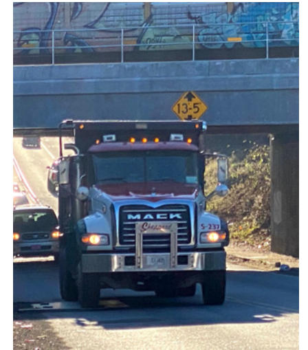
Truck Traffic and Low Bridge Clearance Along Bolton Road is a Safety Concern
