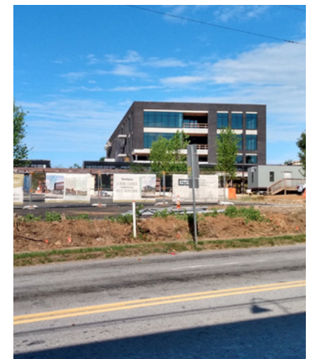
Mixed-Use Development Under Construction on West Marietta Street in May 2022
